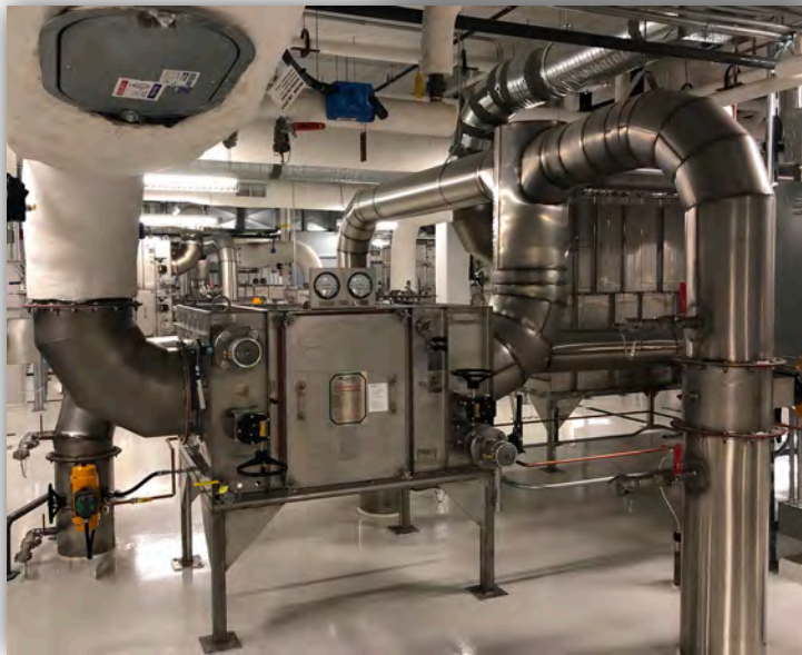
CL3-Ag Animal Cubicle single HEPA filter housing on supply air
