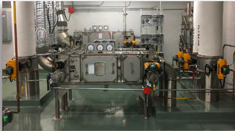
CL3 Lab single HEPA filter housing on exhaust air
