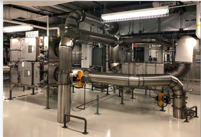
CL3-Ag Animal Cubicle double HEPA filter housing on exhaust air
